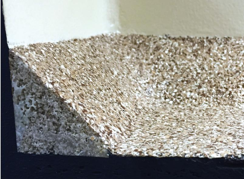
Note there is no 90 degree angle at the wall and floor, the "cove" at the juncture lets water flow away so there is less chance of bacteria build up.
